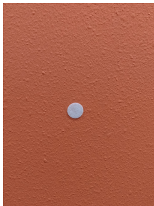
Stick Velcro on wall at equipment location
